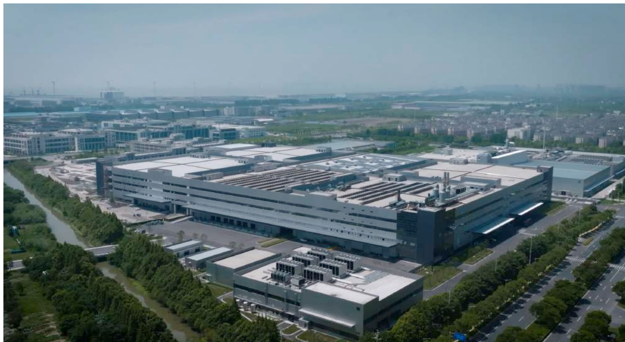
Haiyan Future Factory of the Company
