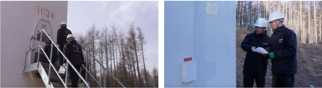
Wind power project site with power cut and technical transformation and upgrading
