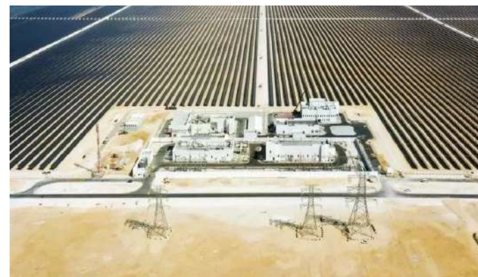
800-megawatt Al Kharsaah PV power station
