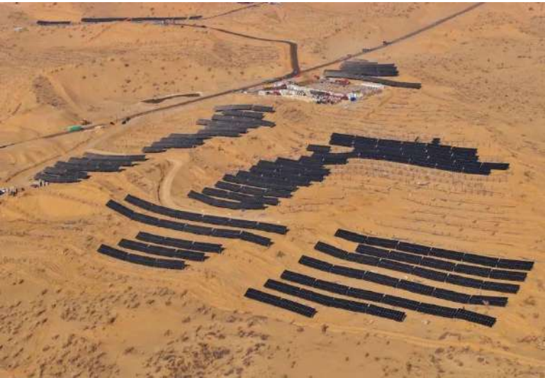
Xinjiang Green Development Midong District 3.5GW PV Project
