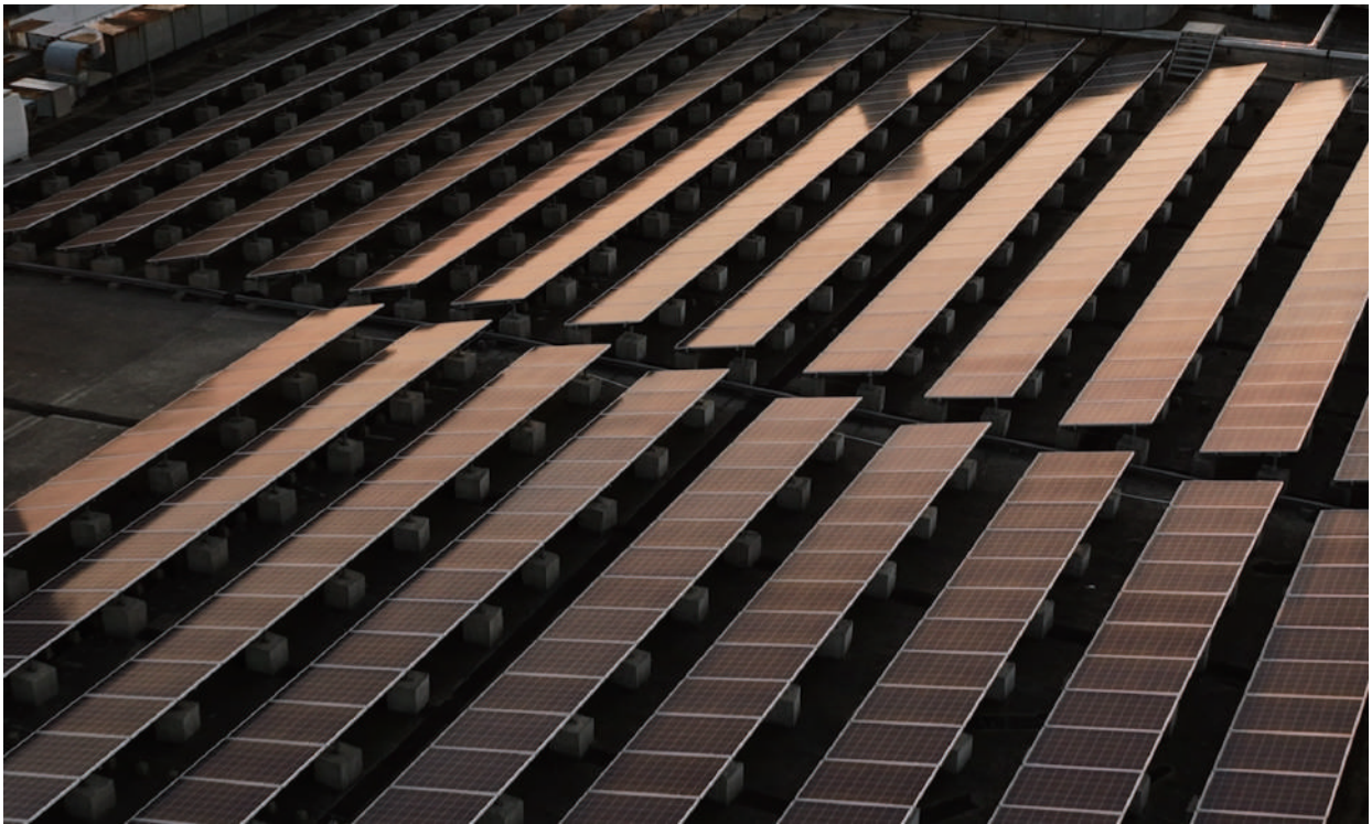
Installation of the distributed PV
